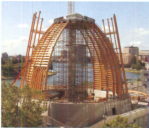
The cathedral structure has inner and outer shells of vertical glue-laminated ribs (left). The inner one, made from curved ribs, takes its shape from the surfaces of a pair of intersecting spheres, while the outer shell is composed of straight elements that define segments of two cones.
