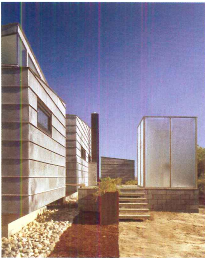
An outdoor shower (left) sits adjacent to the house's main entrance, acting as a beacon at night. A fire pit (below) is made of the same concrete block used for the house's foundation.
