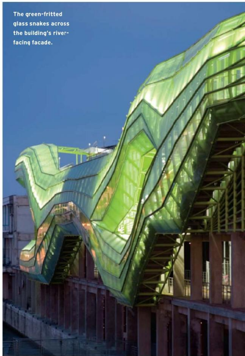
The warped D's and B's of the Plug-Over's structural frame, composed of steel tubes.
