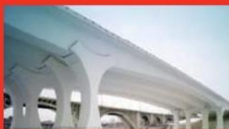
The rebuilt Minneapolis I-35W bridge contains Holcim Envirocore cement.
