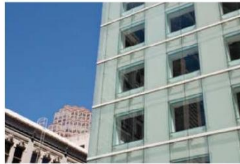
Glass frames span the 9-inch gap between the fritted-glass wall and the original brick facade. Clear glass is used over the existing window openings (above and right).
