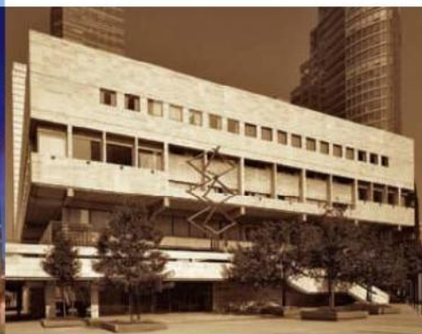
The new expansion and renovation of Pietro Belluschi's 1969 original (left) involved adding a wedge-shaped addition (opposite) with new travertine on West 65th Street, and glazing (far left) on Broadway.
