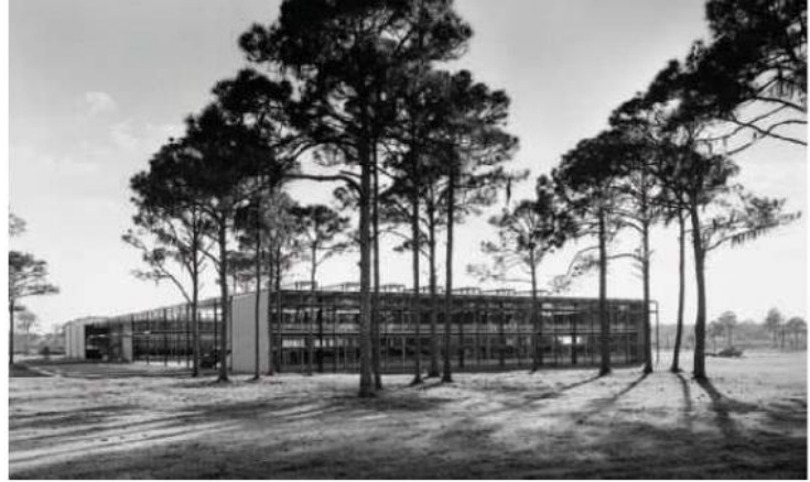
On May 5, the school board approved funds to demolish the building.
