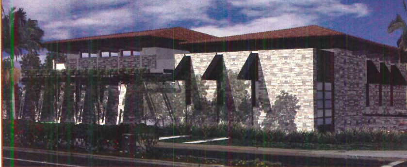
The Westminster, California, Chamber of Commerce building features a barrel tile roof that contributes to LEED Gold certification.
