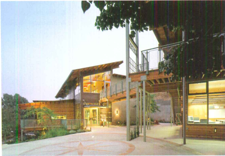
The new library/ student center and classroom buildings are connected by an outdoor commons and catwalklike bridge that transitions into a balcony (left).
