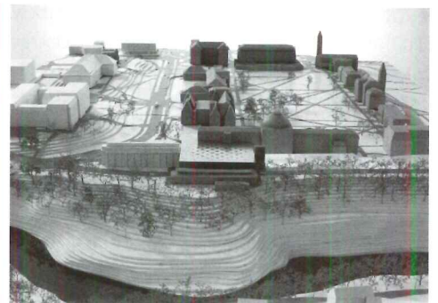
The OMA-designed Milstein Hall will connect two existing buildings on the north edge of the campus Arts Quad (left). A cantilevered, glass-and-steel volume (below left) will extend over a street, toward Fall Creek (below).
