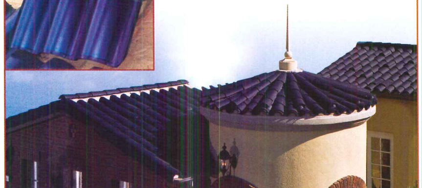
Solar tiles integrate with clay tiles for a seamless look.
