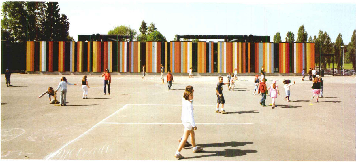
Children play in the courtyard bordered by the new early childhood wing (left). It is brightly sheathed in a rainbow of thin, multicolored fiber-cement panels (left and below).
