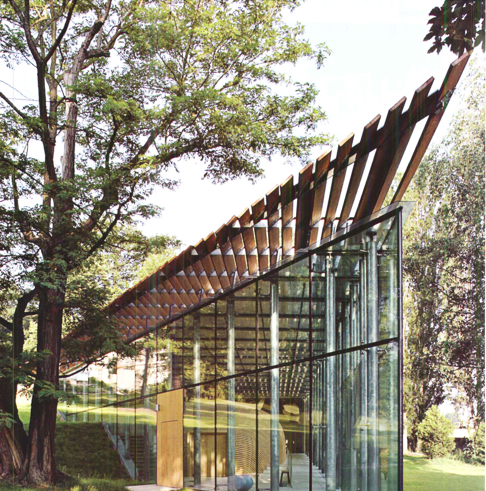
Marc Rolinet's Chapel of the Deaconesses of Reilly emerges out of the hillside as a stark glass triangle (opposite). Its high-tech exterior encloses a handcrafted inner chapel of curved wooden slats (this page).
