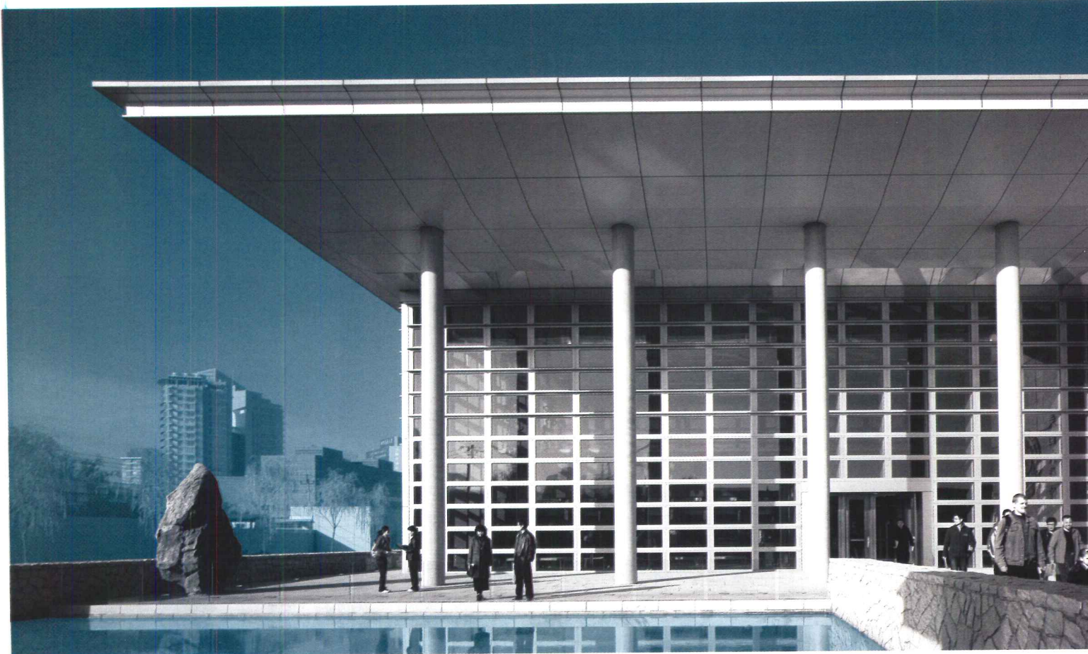
By placing the Beijing embassy behind a protective wall, SOM was able to use lots of glass on its buildings.
