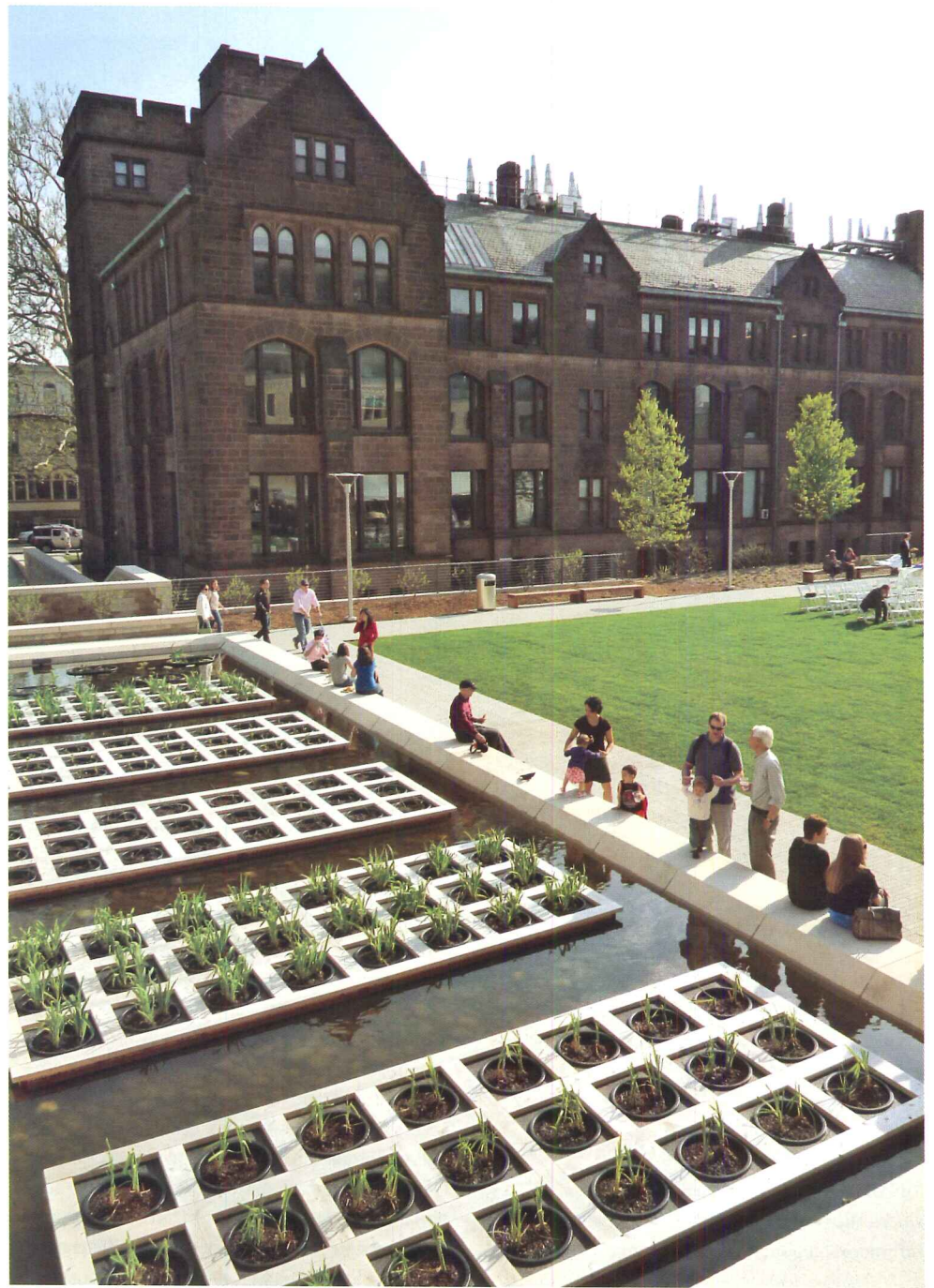
Kroon's runoff cycles through a water feature (right) containing native wetland plants (below) that remove impurities such as nitrogen and phosphates.
