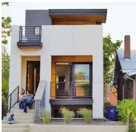
LEFT: This modular, 2,750-square-foot house, on track for LEED Silver certification, was conceived as two boxes that slide over one another to create outdoor living space and a lower covered rear entry.
