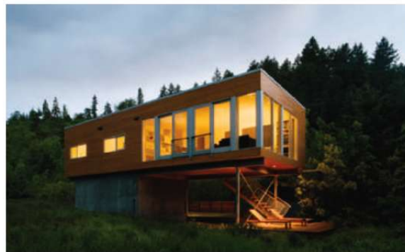
Neal Creek Residence | Paul McKean Architecture | Hood River, Oregon | Submitted by MAIL.
