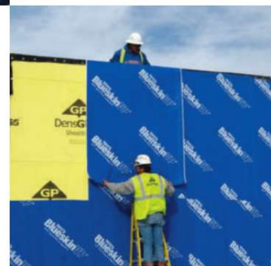
Self-adhering membrane eliminates fasteners that leave holes in the building envelope.
