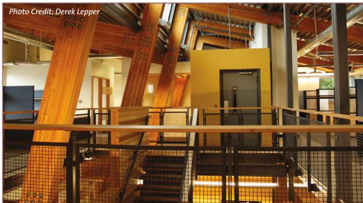
Wood helped the Gulf Island National Reserve Operations center to achieve LEED Platinum status.
