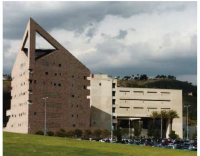
School officials say the building has structural flaws.
