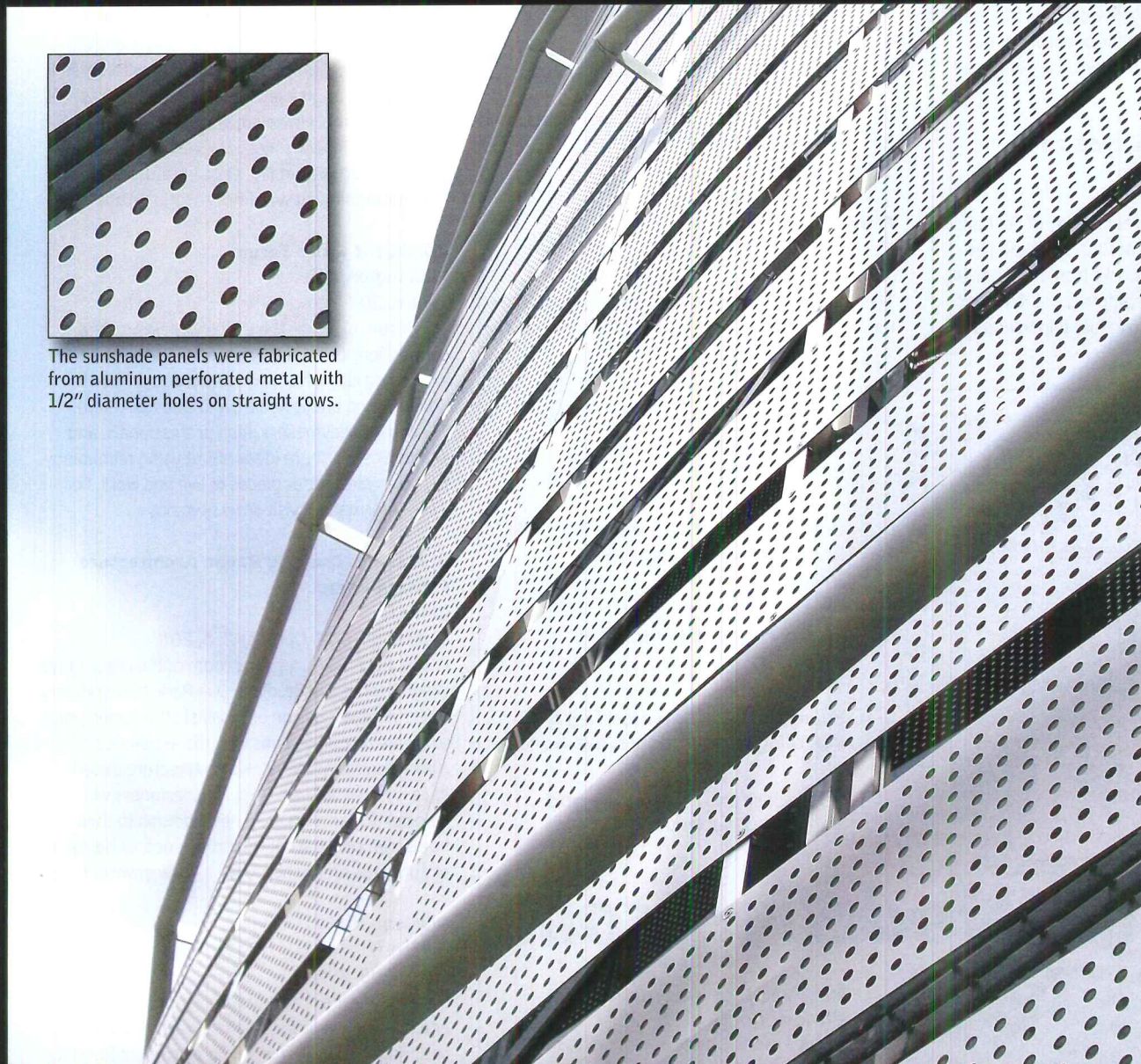
The Barnes Jewish Hospital has an intriguing banded wrap of McNICHOLS ® Perforated Metal panels. The panels act as a sunshade for an addition that houses patients.
