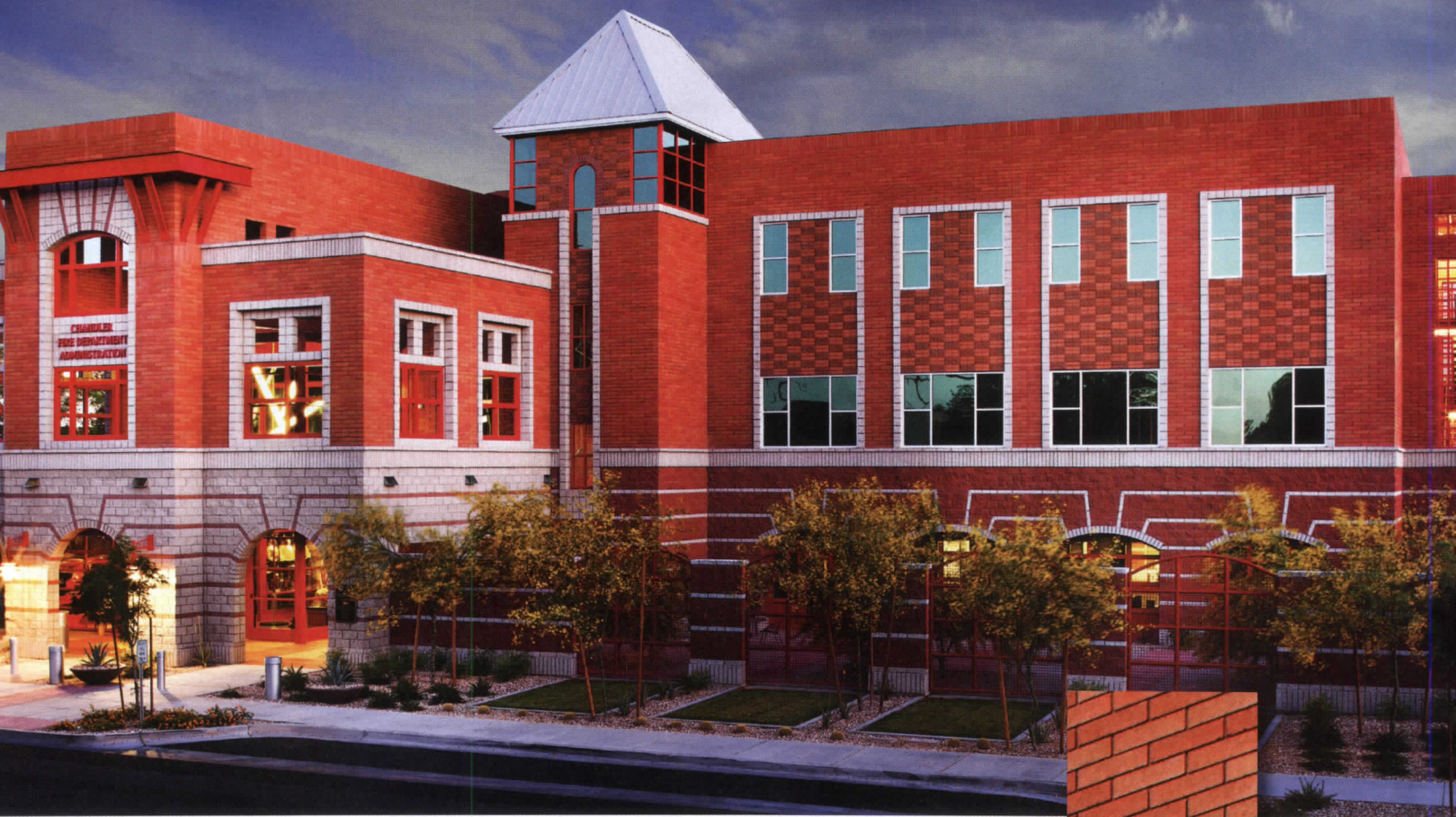
-Project: Chandler Fire Administration Building, Chandler, AZ.
