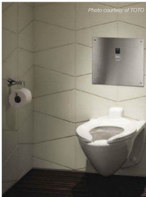
For older population segments, toilets in the universal-height range of about 16.5 inches reduce the effort required to use the fixtures, which helps reduce overall health costs.
