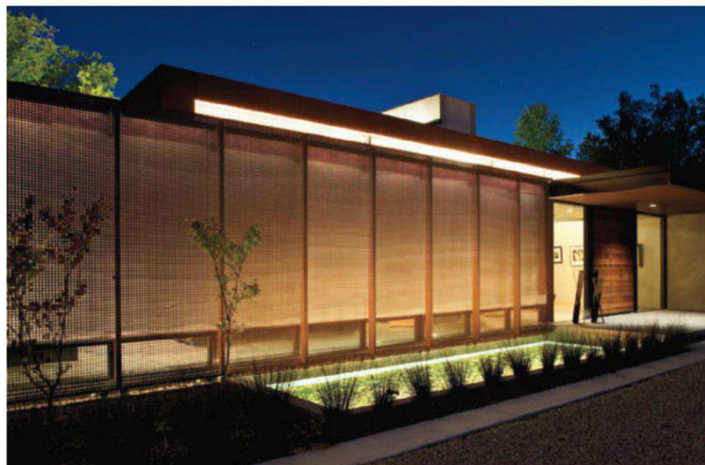
OFF THE GRID Perforations on the metal panels that clad the exterior (left) allow light to permeate the northern (entrance) side.
