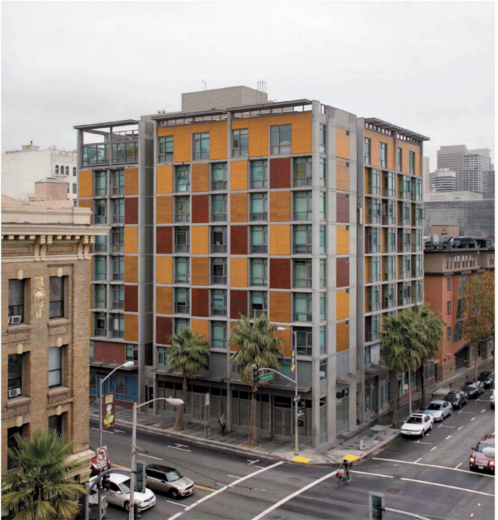
Plaza Apartments. San Francisco, California (U.S.) / Architect: Leddy Maytum Stacy Architects & Paulett Taggart Architects Material: Parklex Facade, high-density stratified timber panels for external use.
