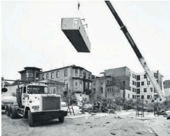
BUILDING BLOCKS The Modules' prefab units took just over four weeks to install (left). The project stands across from a low-rise public housing project and is flanked by brick buildings (below). Signage on the project's west elevation (right) advertises its modular components.
