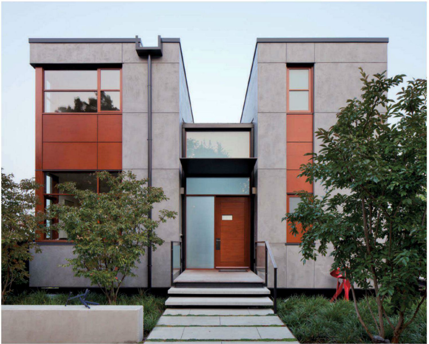
apitol Hill / Balance Associates / Seattle, W.A. / Application: External / Product: Facade / Finish: Copper
