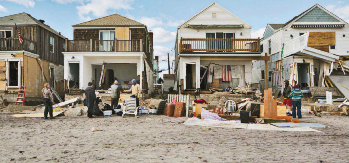
Damaged homes on Rockaway Beach in Queens, New York, after Hurricane Sandy came and went.
