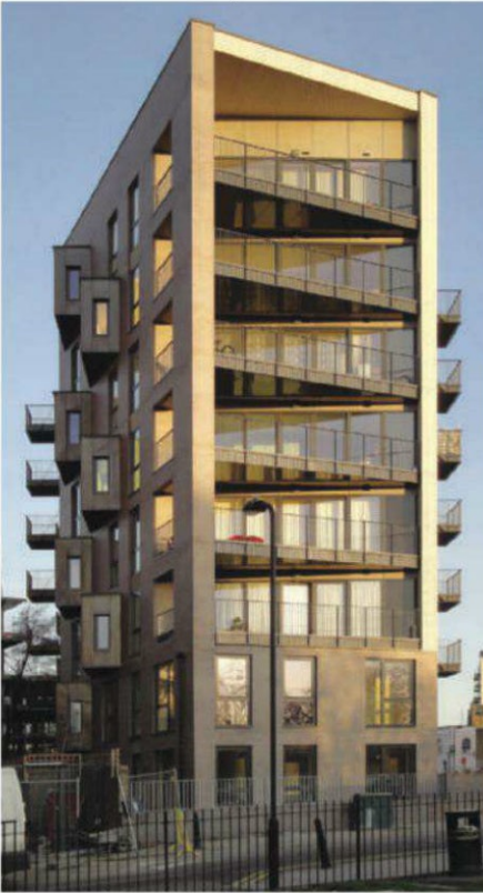
When it was constructed in 2011, Bridport House was the largest timber-built apartment block in the world.
