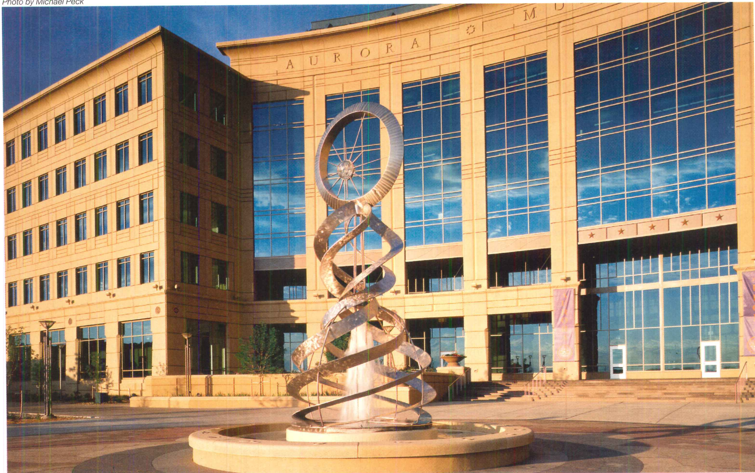
Colorado's Aurora Municipal Building combines open space with a 286,000-square-foot building and a 241,000-square-foot parking structure. Both projects feature total-precast concrete structural systems, which combined architectural and structural components into single units.
