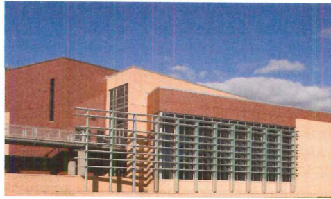
Fixed exterior shading devices like the ones shown here cannot adjust to changing weather and light conditions.
