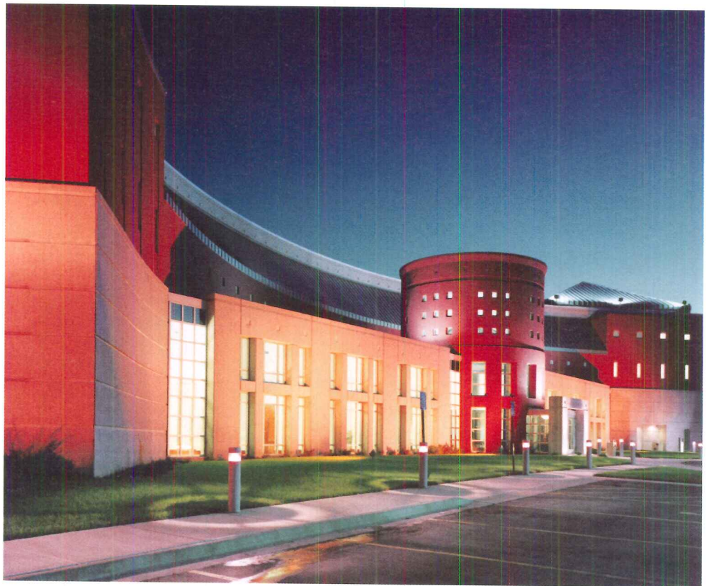
Properly designed EIFS meet all of the building code requirements for using foam plastic insulation in exterior walls.
