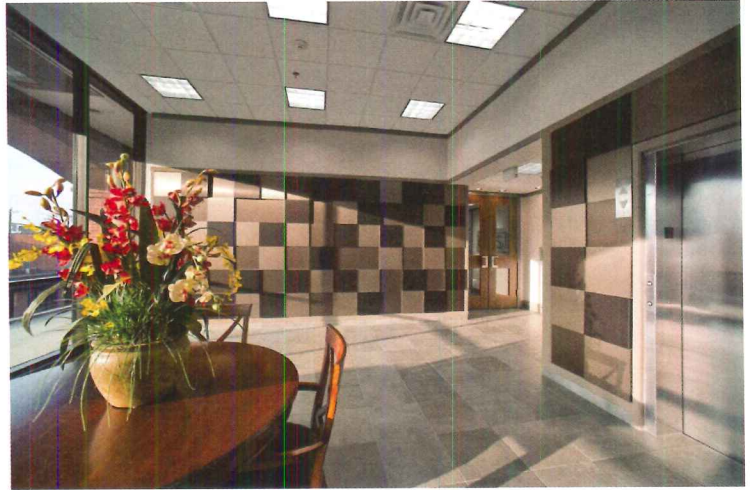
Left: Anodized aluminum in a clear matte finish was specified for sunshade louvers at the Winspear Opera House, Dallas, Texas. Right: High-pressure laminate anodized aluminum may be used for interior walls with multiple colors.
