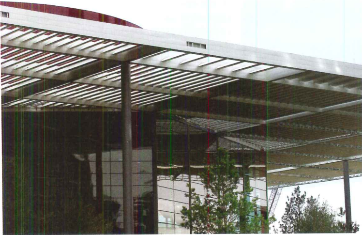
Left: Anodized aluminum in a clear matte finish was specified for sunshade louvers at the Winspear Opera House, Dallas, Texas. Right: High-pressure laminate anodized aluminum may be used for interior walls with multiple colors.
