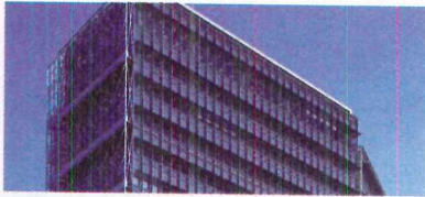
Daylight Autonomy 101 Sponsored by Lutron Electronics Co., Inc. Photo courtesy of Coscia Moos Architecture
