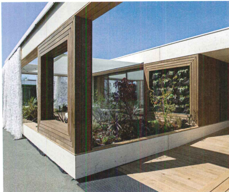
TEAM AUSTRIA, VIENNA INSTITUTE OF TECHNOLOGY Flexible design was the key tenet of the first-place winner—it can be built as a stand-alone residence or as a component in a multifamily design. Triple-glazed walls and an automated screen and awning system keep out heat while letting in plenty of sunlight at the right time of day. In the bath, a shower tray that recovers heat cuts the demand for hot-water heating by roughly a third. A gracious wooden ramp forms a welcoming and accessible entryway.
